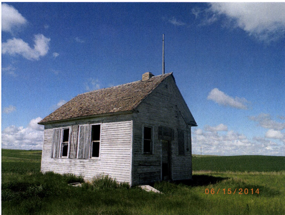
Figure 3: View of MAC-MNB-2002, to the southwest (Image 2621).
