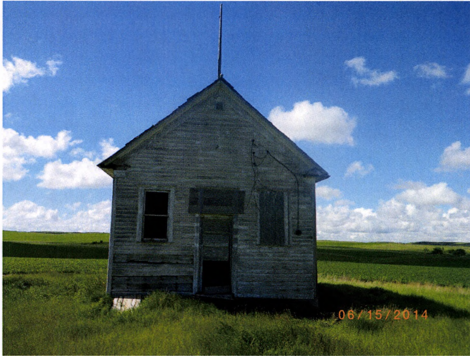
Figure 2: View of MAC-MNB-2002, to the south (Image 2630).
