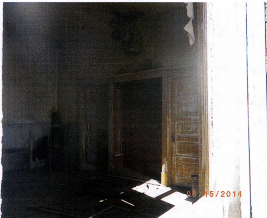
Figure 5: Doors from entryway into school (Image 2638).
