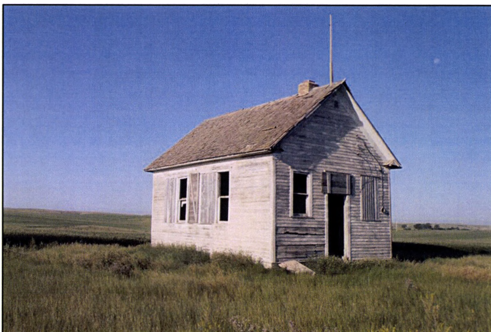
Site facing southwest.
