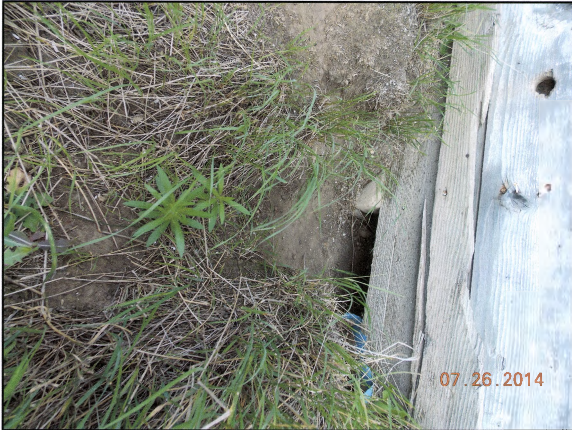
Figure 10: Close up of the stone and concrete footings for the structure.
