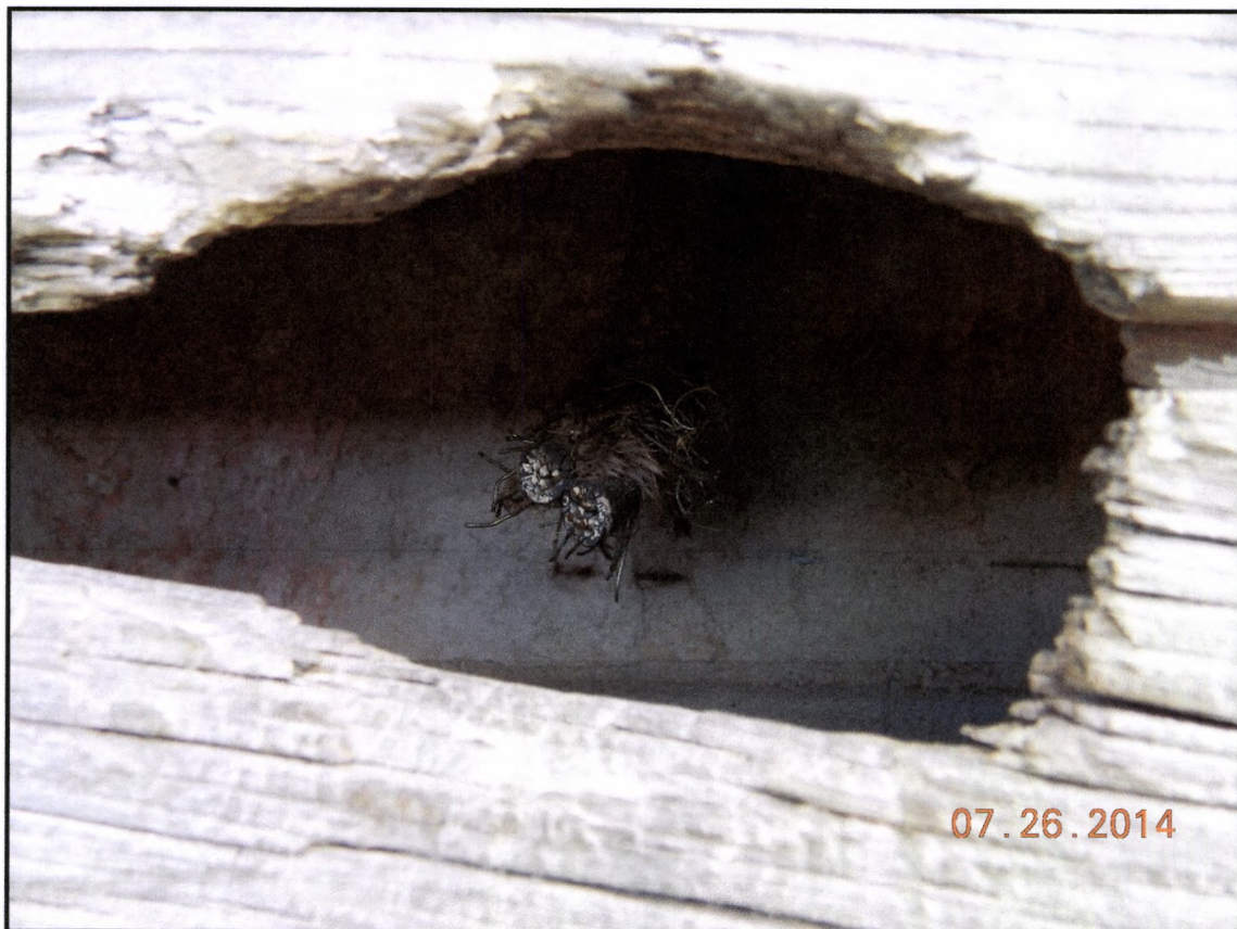
Figure 9: Close up of conduit showing that the schoolhouse had electricity at one point.
