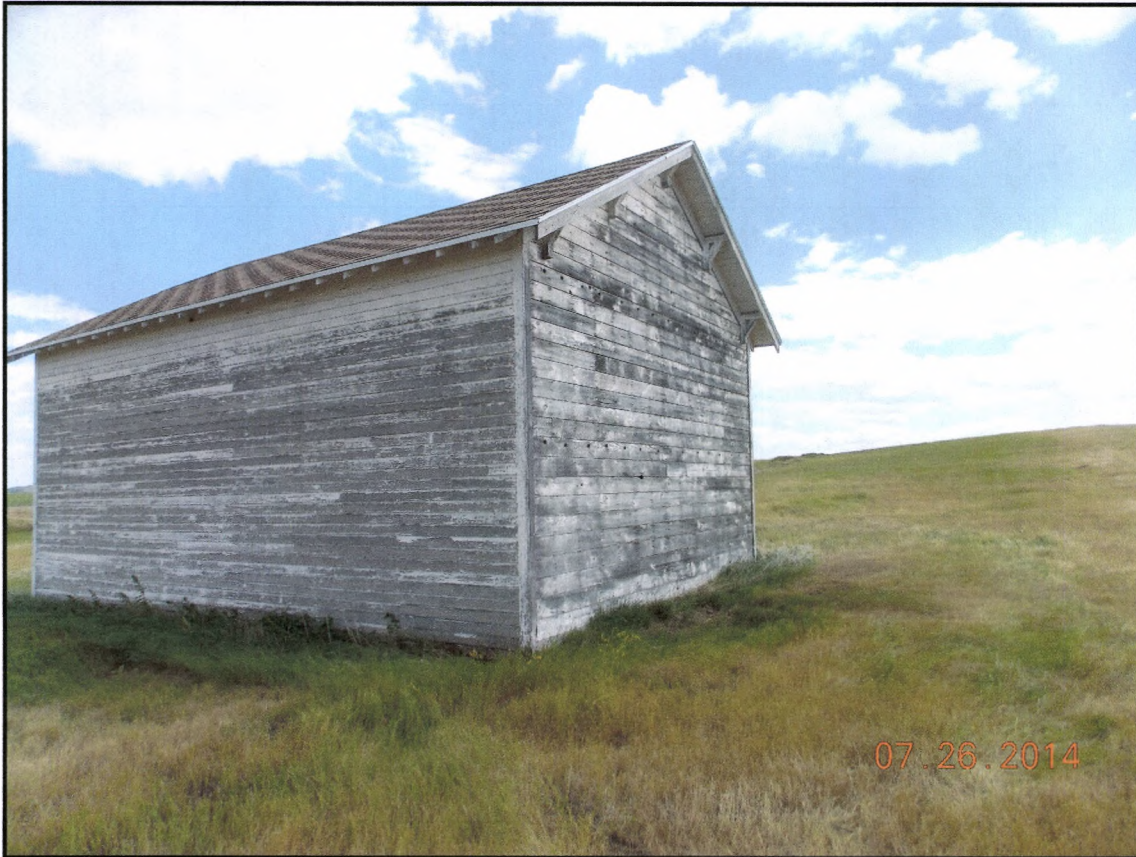
Figure 6: Overview of schoolhouse facing southeast.
