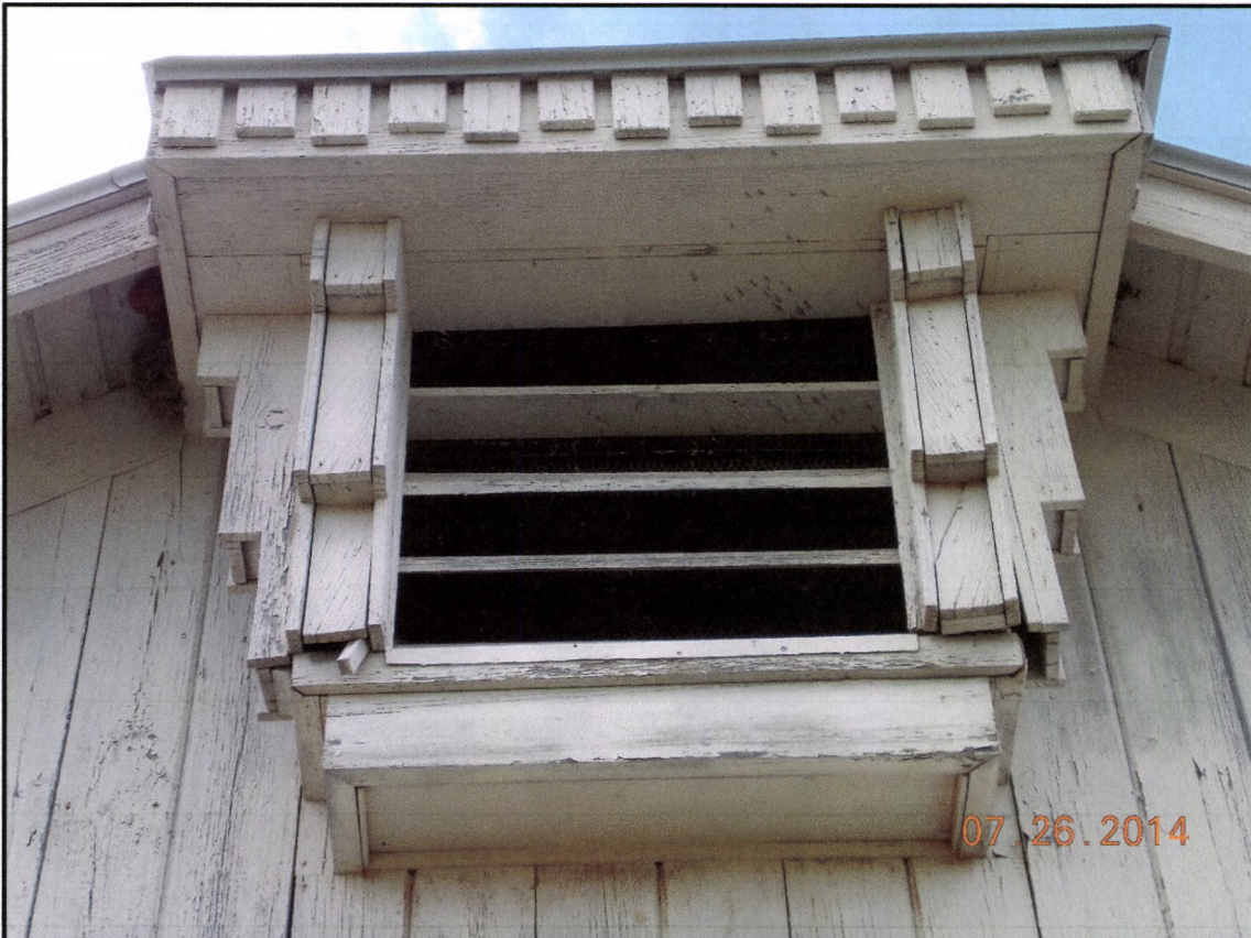
Figure 7: Close up the ventilation window below the hip and above the entrance to the schoolhouse. Review by Bleier in 2016 indicated that this type of vent is relatively unique.
