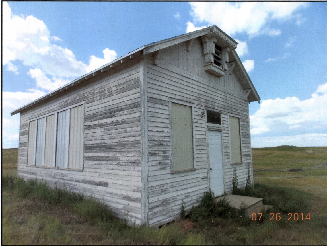
Figure 4: Overview of structure facing northwest. The decorated vent and the hip of the roof noted by Amy Bleier in 2016 are in the foreground.
