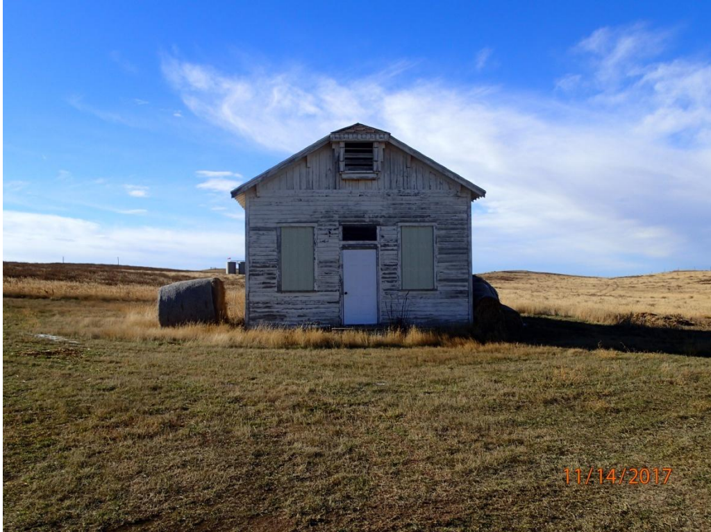
Figure 2: Site 32MZ3004 overview, looking to the west.
