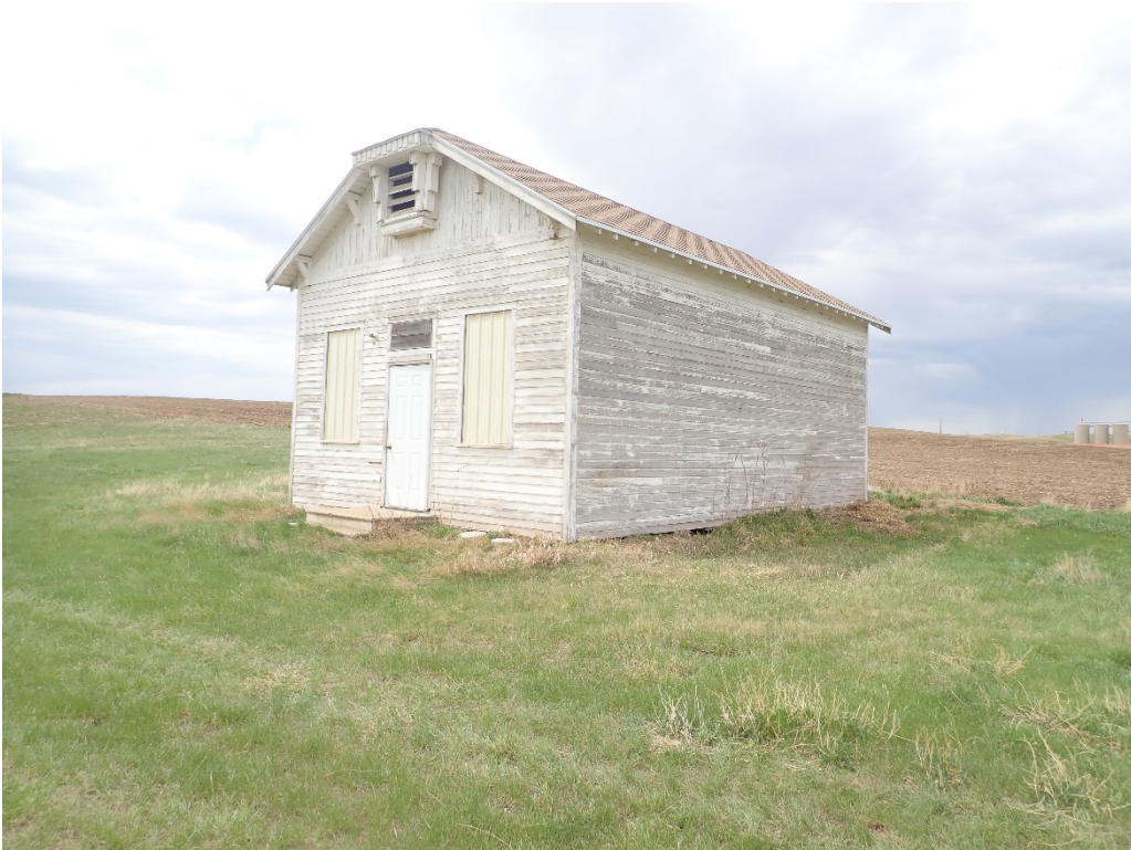
Figure 4. Site 32MZ3004, facing southwest.
