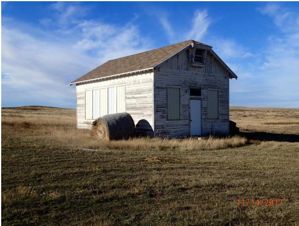
Figure 1: Site 32MZ3004 overview, looking to the northwest.
