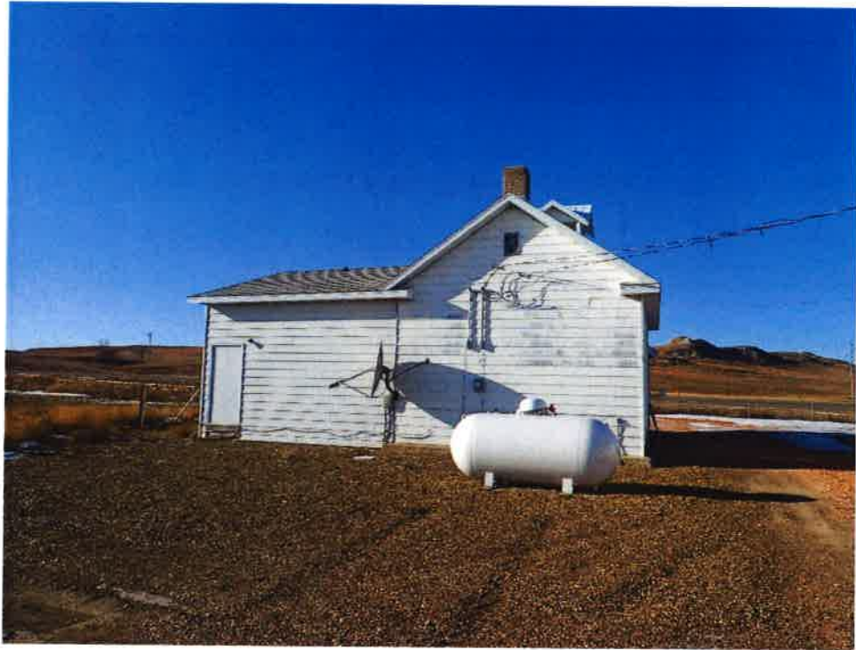
Figure 5: Feature 1 looking west, January 10, 2020.
