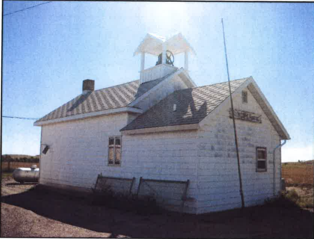
Figure 4: Overview of Feature 1, the School, showing the northern and western elevations.
