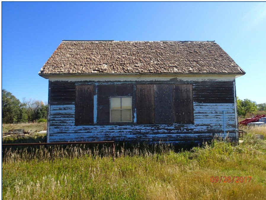
Figure 4: Overview of BCA17-1064-Site3 Feature 1. View is to the east.
