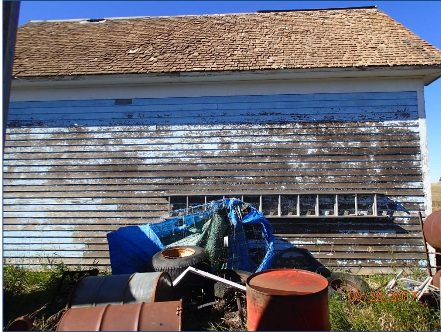
Figure 3: Overview of BCA17-1064-Site3 Feature 1. View is to the west.
