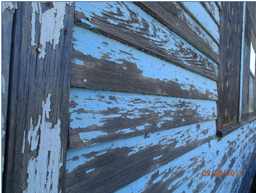
Figure 6: Close up of siding on northwest side/corner of BCA17-1064-Site3 Feature 1.
