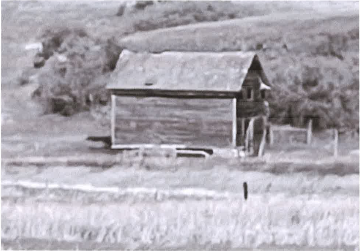
Northwest Side and Southwest End
