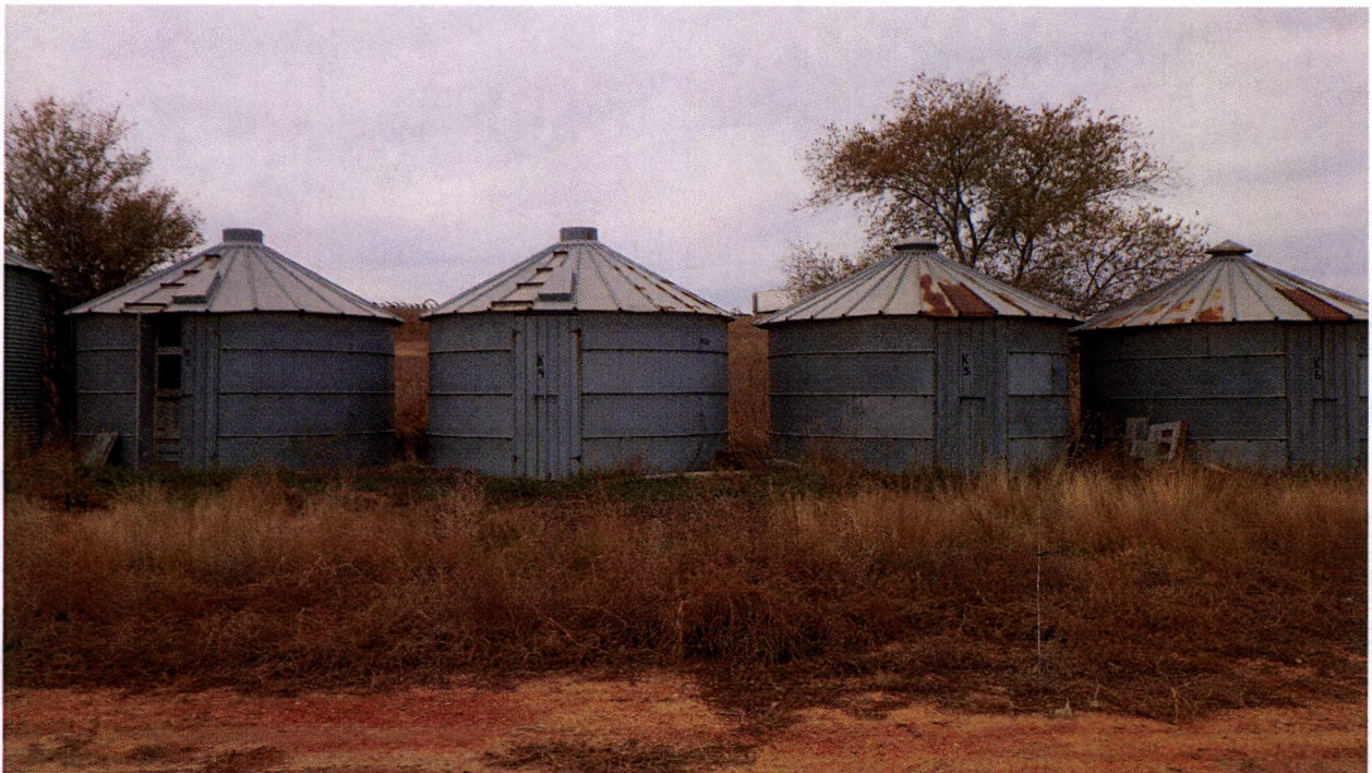
Figure 6: MAC-NKL-56x, Feature 4 (left) and Feature 5 (right), view east (Image 5618).
