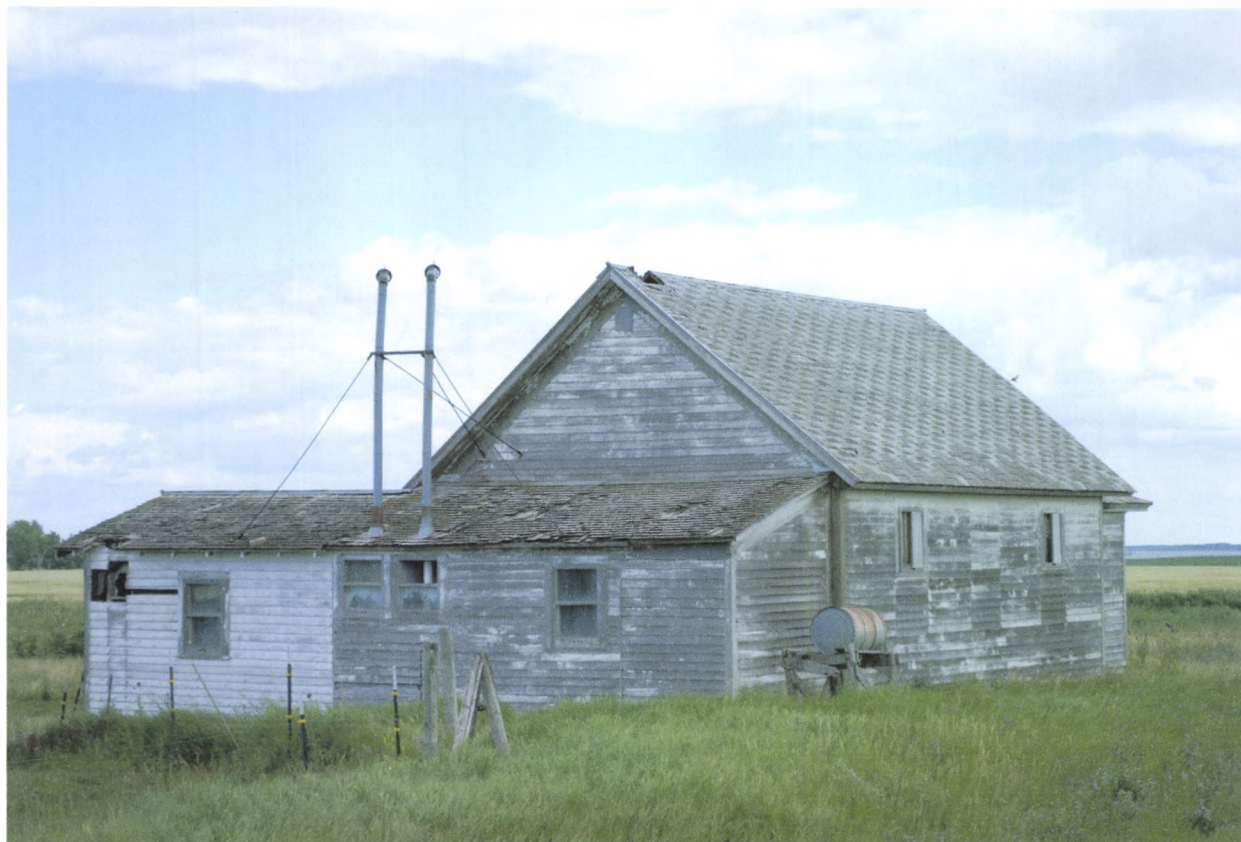
Feature 1 northwest corner
