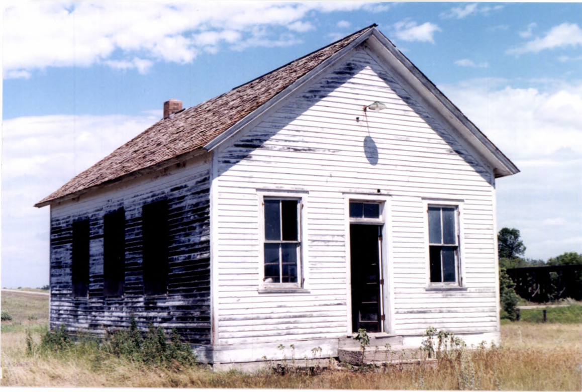
Feature 1, view from the southwest.
