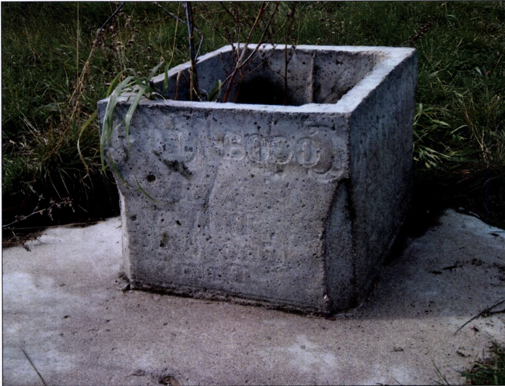
F3 concrete platform, detail (79F13-071).
