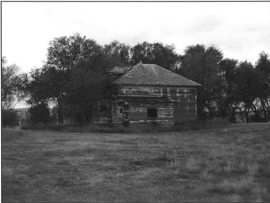
Overview of the standing schoolhouse (view SSW; 79F-018).
