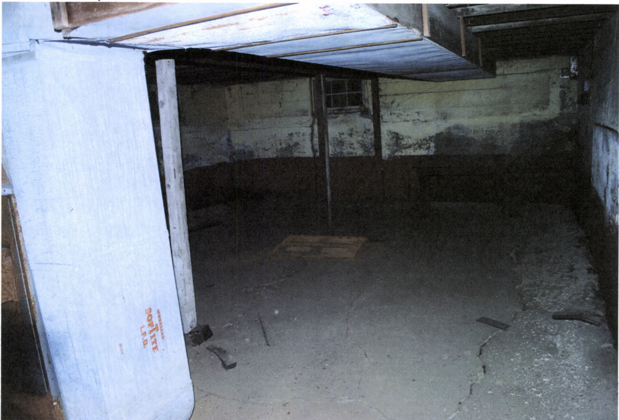
Danton School, interior basement, west wall
