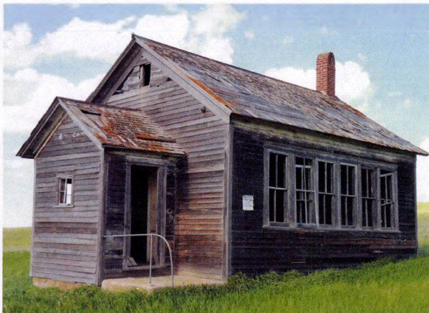
April 19, 2011 view to northeast of south and west elevations.
