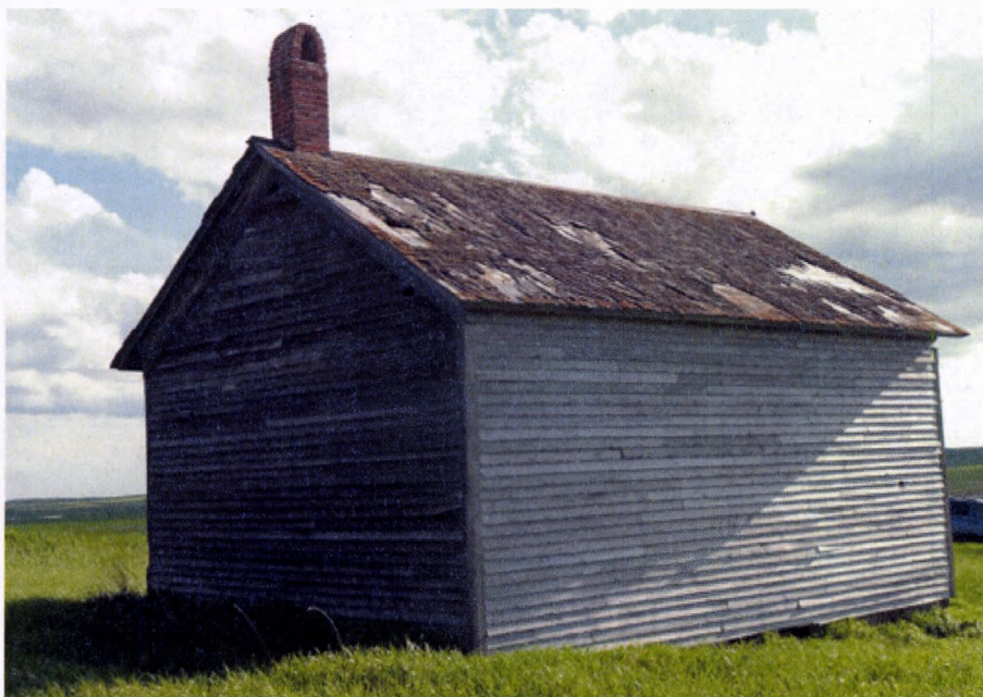
April 19, 2011 view to southwest of north and east elevations.
