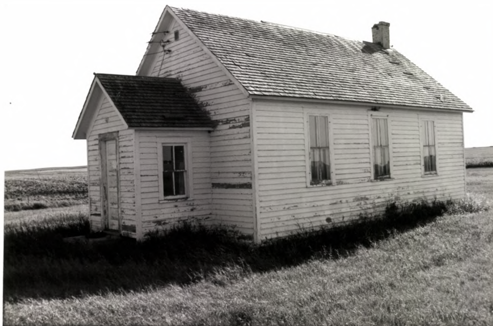
6:12 SCHOOLHOUSE FROM THE NE
