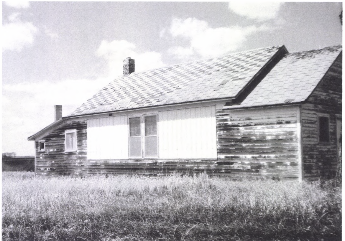
South Side (and all you can see of the East!)
