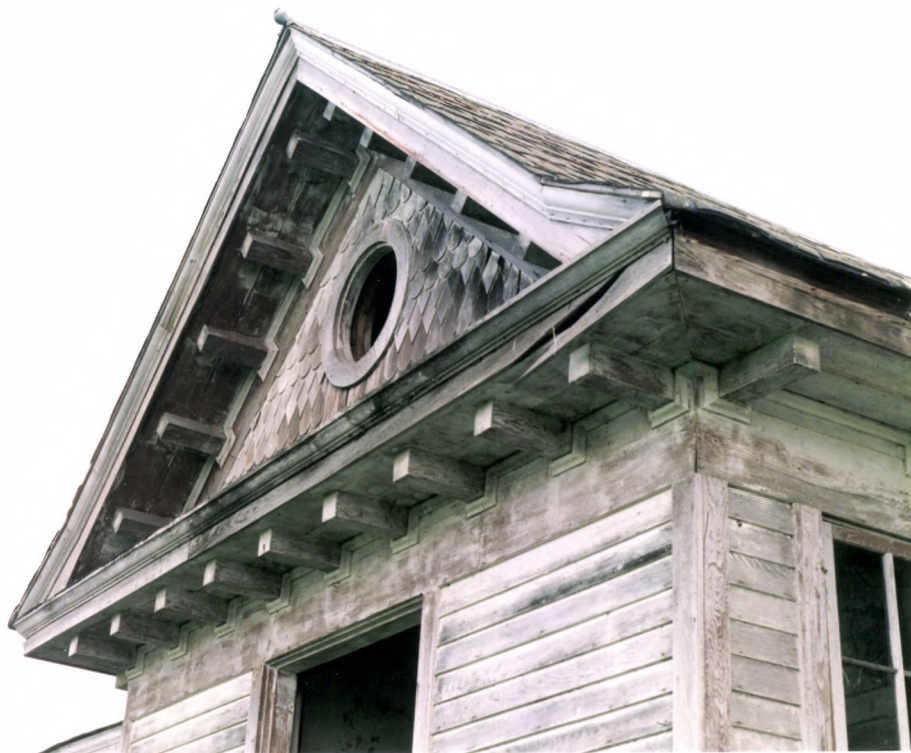
Feature #1, vestibule pediment detail, view from northeast, roll 1, frame 30.
