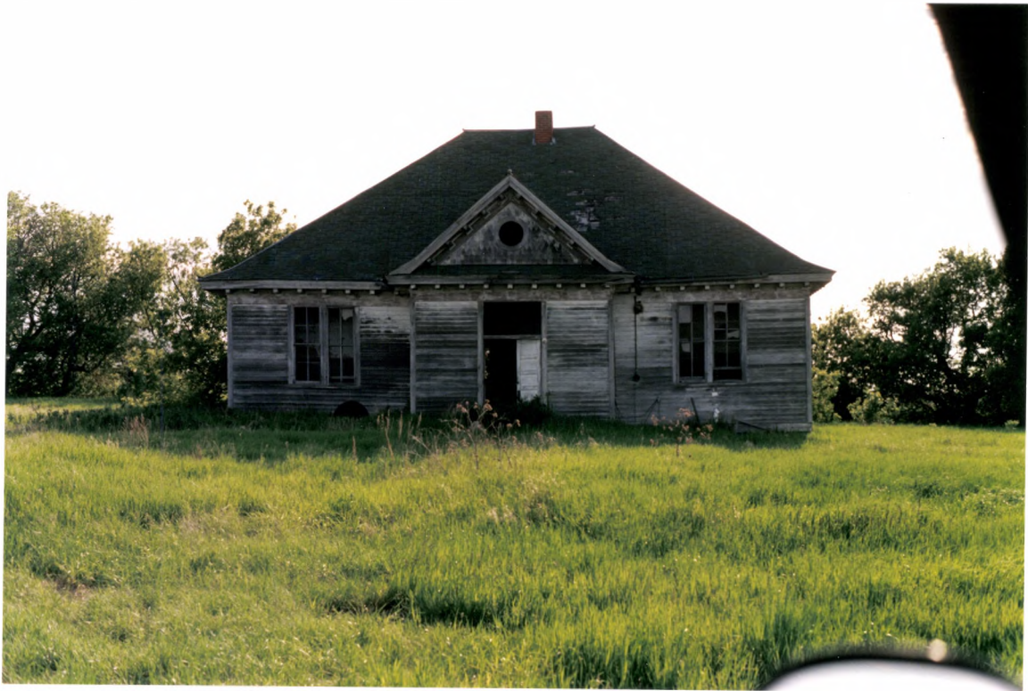
Feature #1, view from east, roll 1, frame 27.
