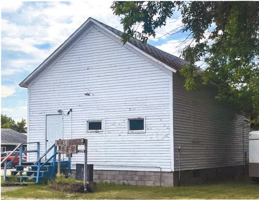
North Side and West Side (Right side of the picture)
