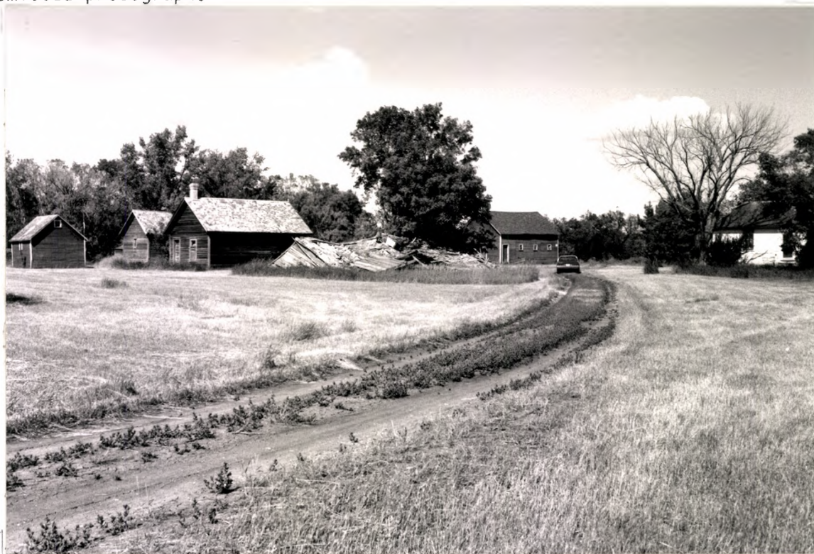
ABOVE: BW1-1 Acton townsite (Hoenke farmstead), 32WA7. View NE of farmstead. Abandoned house to right. Fallen structure reported to be original town building. July 17, 1990
