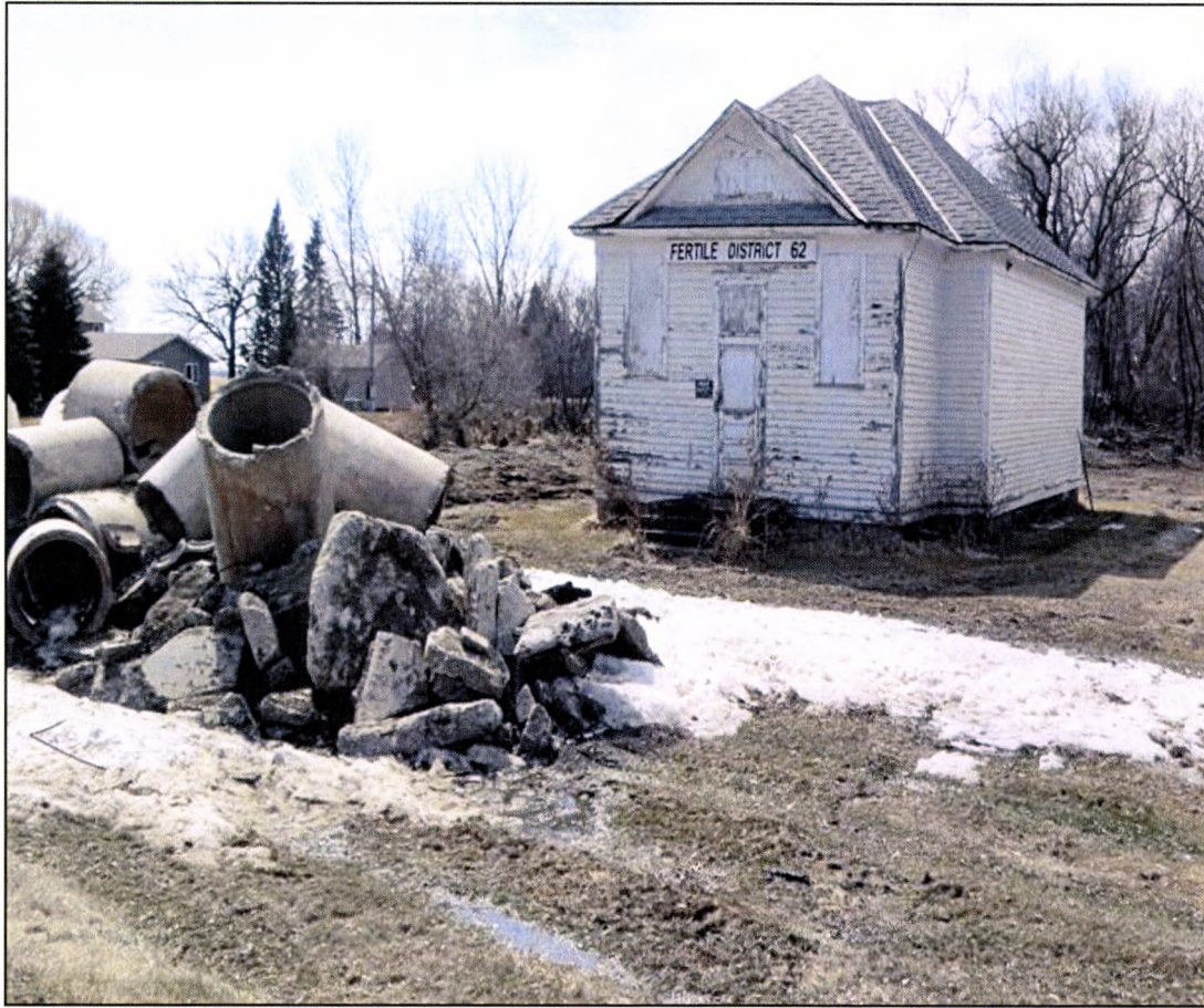
Figure III: Side view of Fertile Valley Schoolhouse, note construction debris.
