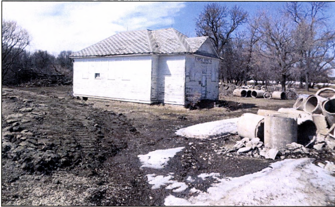
Figure 1: Side View of Fertile Valley Schoolhouse, note construction debris.
