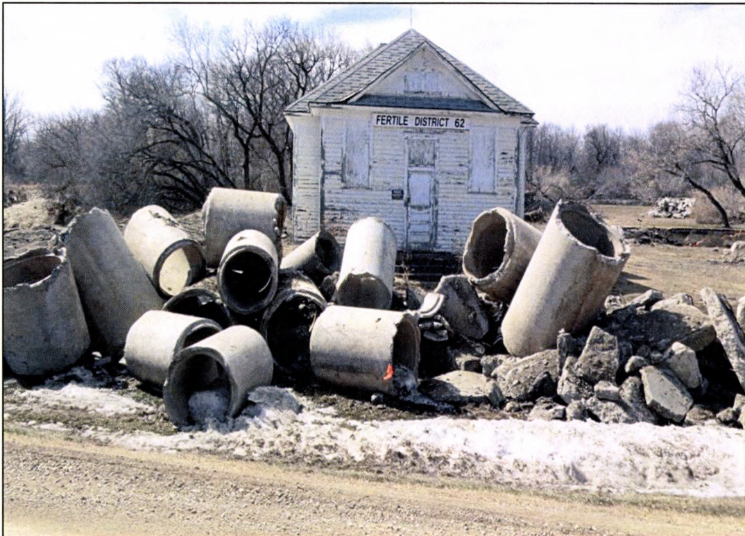
Figure II: View of Front of Fertile Valley Schoolhouse, note construction debris.
