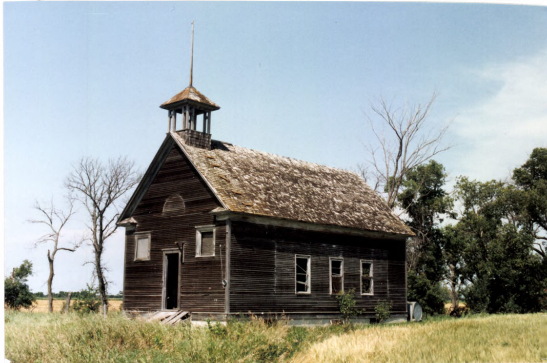
Southeast corner of the school house, view northwest. LP95-CP308.
