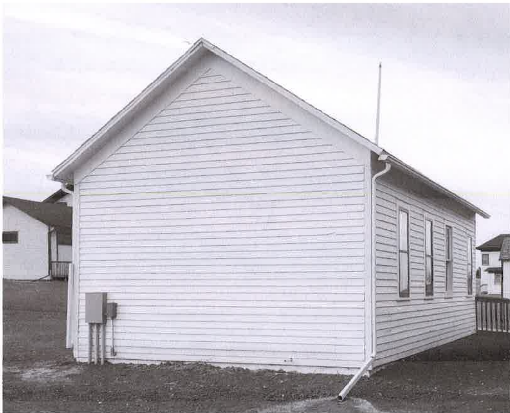
Southeast and North East Side
