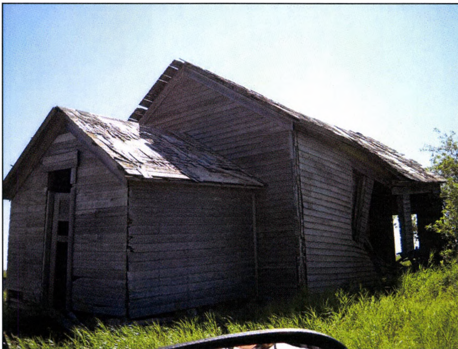
Figure 2: Southwest view of feature (Image #015).
