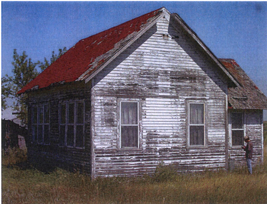
Figure 1: View of school/church to the northeast (Image #1894).
