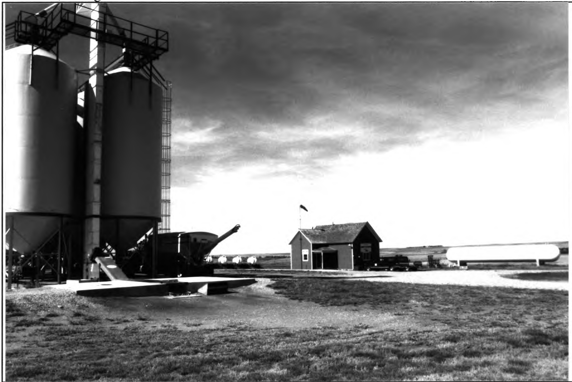
Overall View, facing NW
