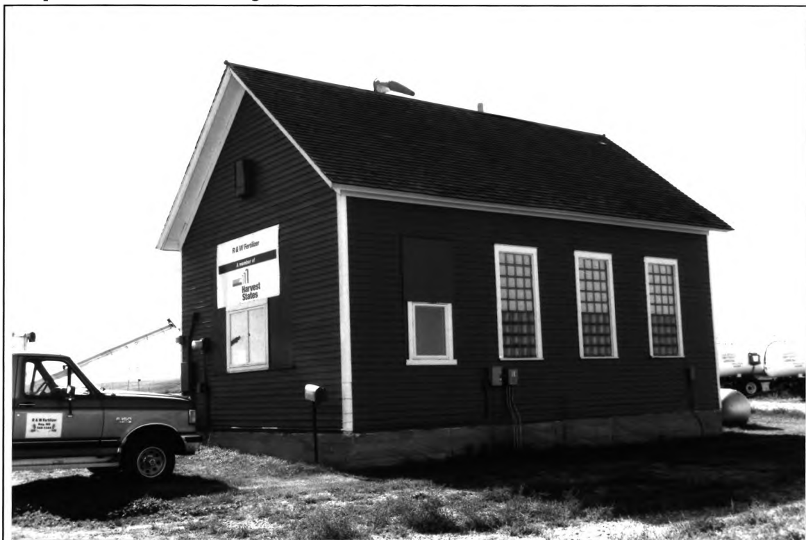
Township Hall (Feature #1), facing SW
