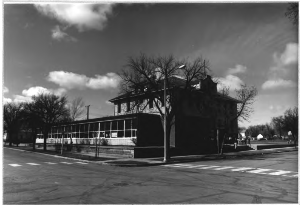
FEATURE # 1 ROLL 6 FRAME 19 view to NW
