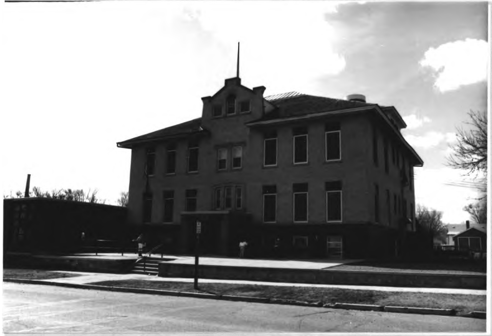
FEATURE # 1 ROLL 6 FRAME 21 view to SW
