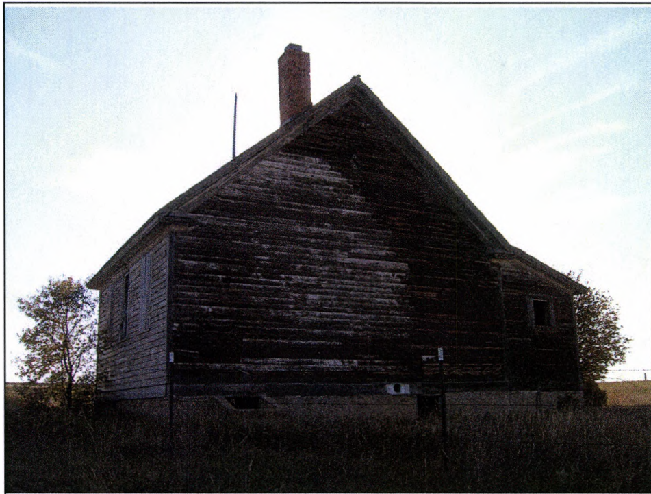
Figure 4: Feature 1, view to southeast (Image #818).
