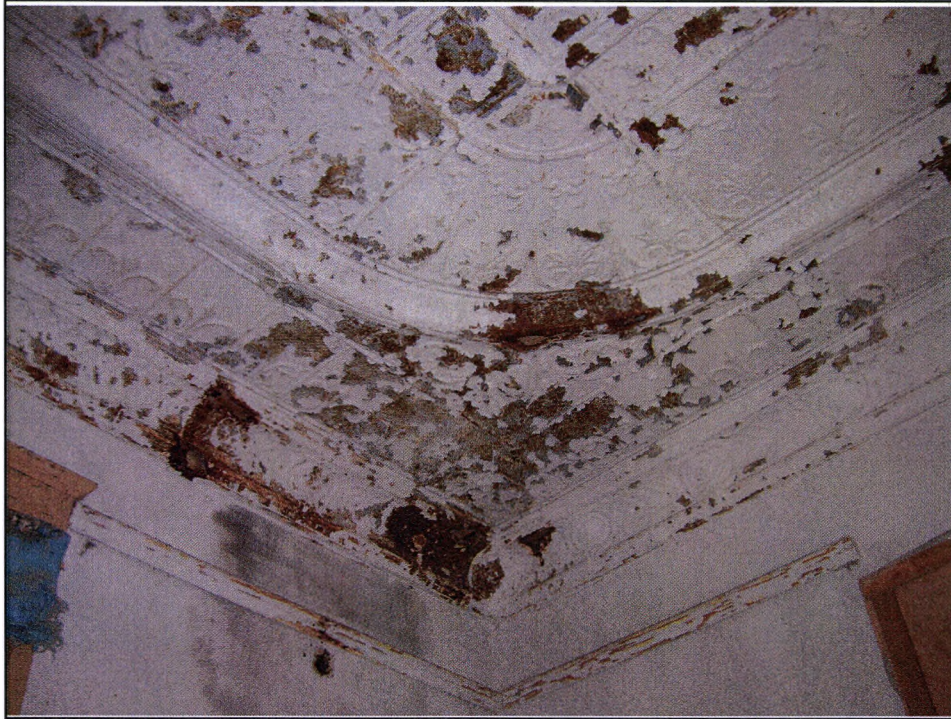
Figure 4: Feature 1, interior sample of the pressed metal ceiling (Image #832).
