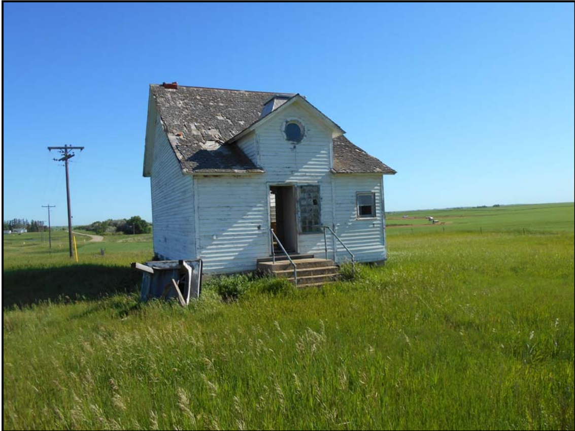
Figure 4: Overview of Feature 1 facing northeast.
