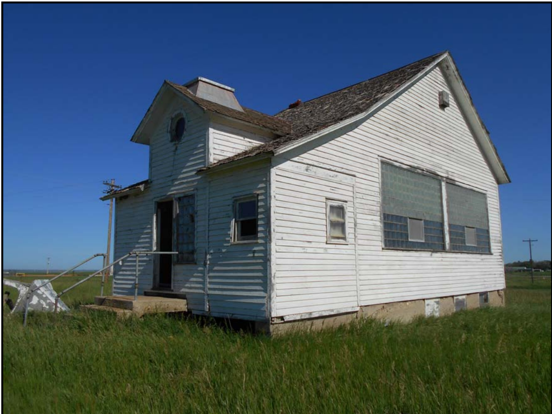
Figure 7: Overview of Feature 1 facing northwest.
