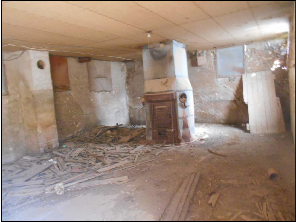
Figure 8: Overview of the furnace in the basement of Feature 1.
